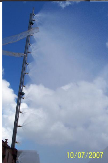
Installation of spray booms at base of gantries
