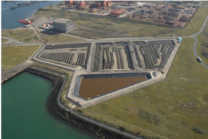
Figure 14 : Dredged treatment platform
